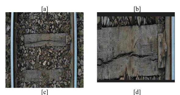
Figure 1. UAV imaging investigation of the station's track: a) an image of a track segment, and b), c), and d) subsequent enlargements of the image of this track segment.
